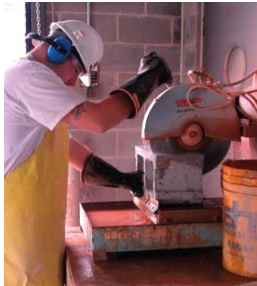
Correct way to cut masonry.
